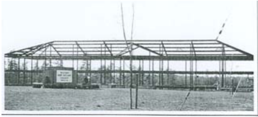
Construction of West Building, 1963 (now Herman Hall).
